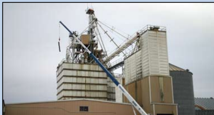
A crane lifts equipment that helps put the finishing touches on the new pellet mill installed at the feed mill this winter.
